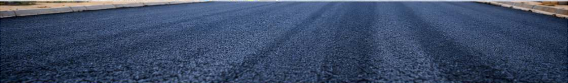
ASPHALT OVERLAY FROM PANSHEKARA TO MADOBI ROAD
